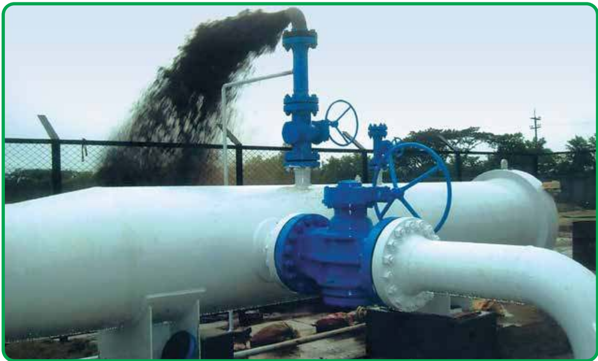
Hydrostatic Test of Anwara-Fouzdarhat Pipeline
